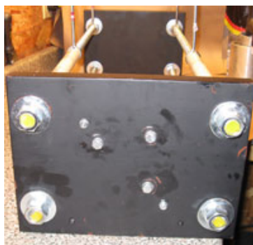
Attachment Holes, Bolts and Nuts in Bottom Steel Plate
