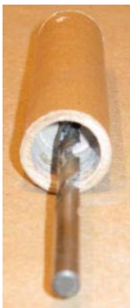
Hand-Twist Drilling a Passfire Hole through Clay Bulkhead
