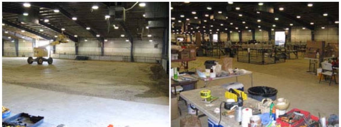
An Empty Room Transformed into a Pyrotechnic Playground
