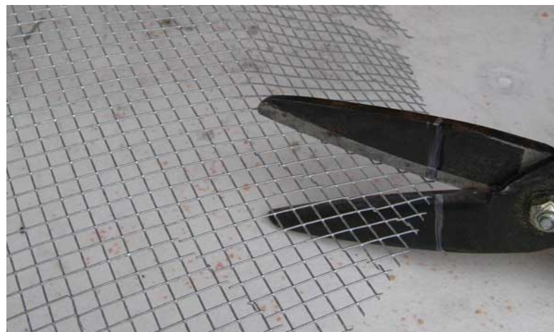
2-1/2" Long Slices Cut into Edge of Screen
